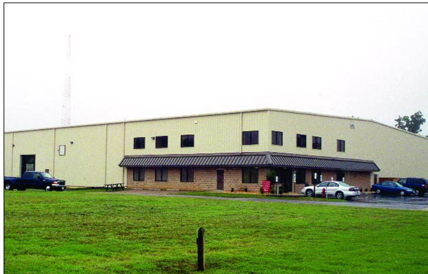
The new 50,000 sq ft Central Marketing, Inc. training and remanufacturing center in Prince George, Virginia.
